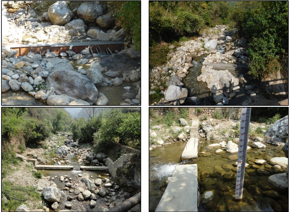
Fig. 3. 1: Various phases of construction of Weir at Henval
